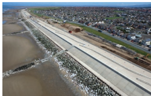
Figure 5: Coastal defences in construction at Rossall, 2017. Photo: © Wyre Council/Balfour Beatty Civil Engineering Ltd.
