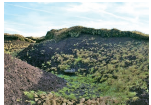
Figure 5: Gullies blocked by stone dams. These stabilise the gully floors, promoting re-vegetation and helping to raise water tables. Photo: © Moors for the Future.
