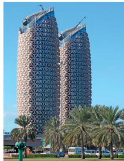
Figure 3: The sunshades on the Al Bahr Towers in Abu Dhabi open and close according to sunlight levels. Photo © Philip Lange/ Shutterstock.com.
