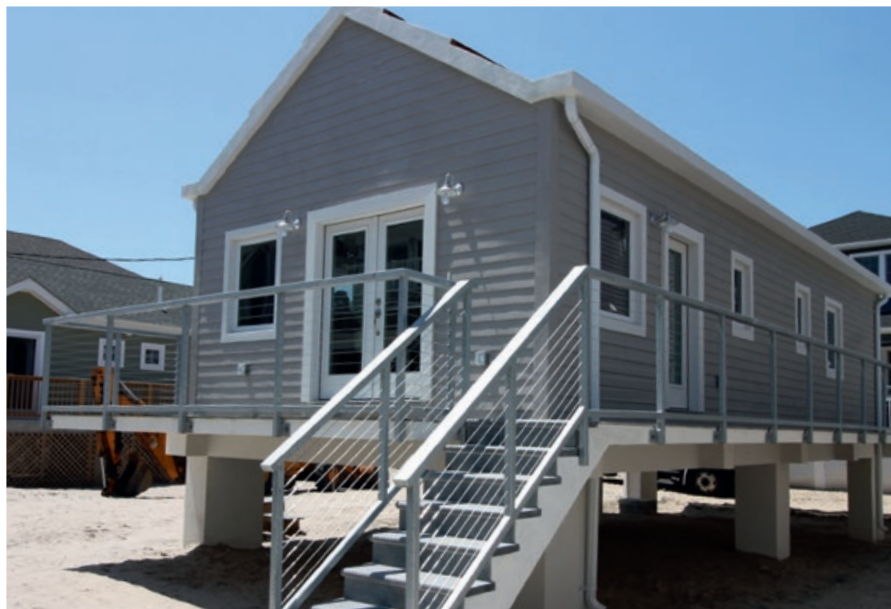
Figure 2: This flood-proof house uses concrete stilts to raise it above likely high-water levels. Photo © Architect Jorge Fontan AIA, Fontan Architecture.
