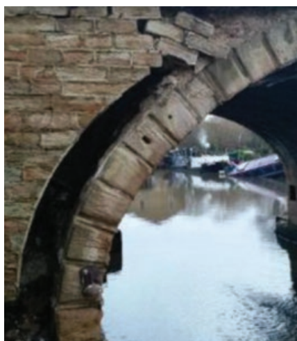
Figure 1: The strength of the flood cracked the bridge at Elland. Photo © Canal and River Trust.
